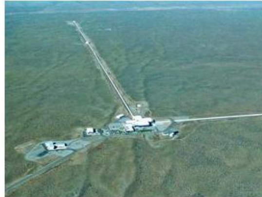
The project of Ligo India will not just help a new generation of physicists, but it will also bring precision engineering to the Indian industry.
